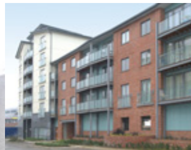
Left: A six-storey timber framed housing development.
