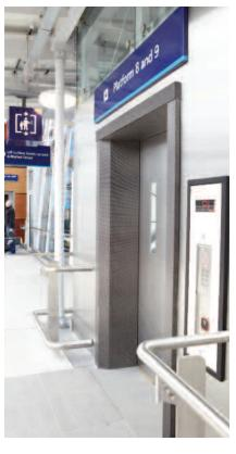
The new 33-person, Network Rail specification, 2-floor semi-scenic hydraulic lift serving platform 8/9
