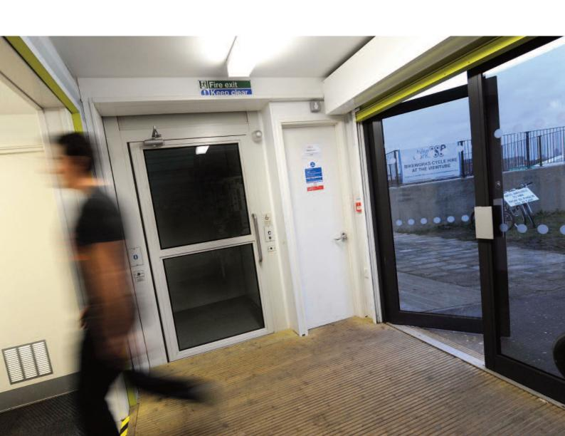
Supplied within a structure-supported enclosure, the Midilift SL does not require a purpose-built lift shaft or lifting beam, so installation was straightforward, taking just five days from fitting to commissioning. Simple and safe to operate it has a rated load of 400kg (4 persons). The platform is controlled by constant pressure buttons and has a maximum travel of 5m at a speed of circa 0.08m/s.
