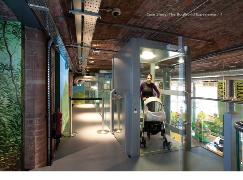
"As specialists in 3D design solutions for every variety of commercial environment, we are used to resolving a project's unique challenges. The BugWorld Experience's vaulted ceilings created a height-restriction issue which determined the type of lift required. Not only did the Stannah Midilift's lifting mechanism fit in neatly, but the lift also provided the most overall costeffective solution."
