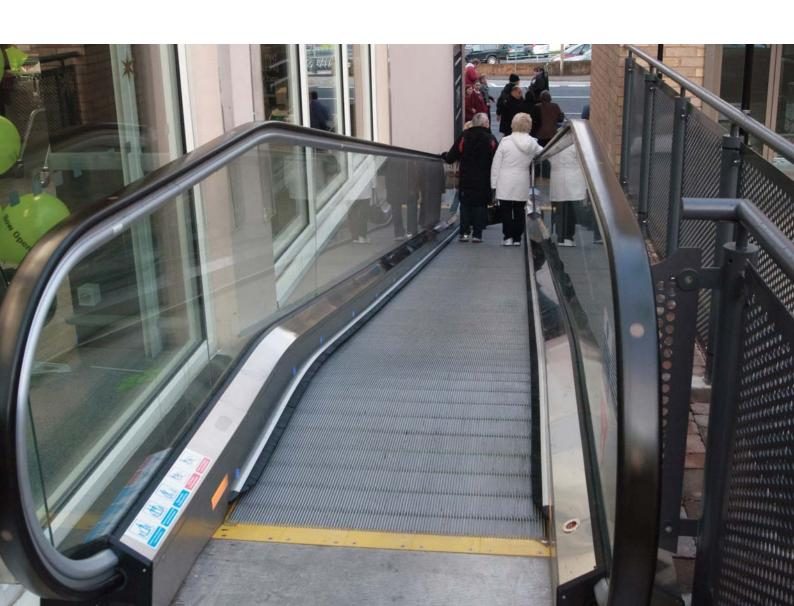
"Our external moving walkway at 5Rise offers full outdoor protection utilising galvanisation and corrosion-proof materials. Internal heaters are also installed to help maintain optimum performance in winter conditions. Because site access was in an outdoor, open environment we could fully assemble the machine in our factory and deliver it swiftly to site fully built and ready for the heavy duty job required of it – moving up to 9000 pedestrians per hour."
