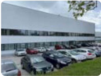
New factory in Brno with a production area of 5,300 m 2
