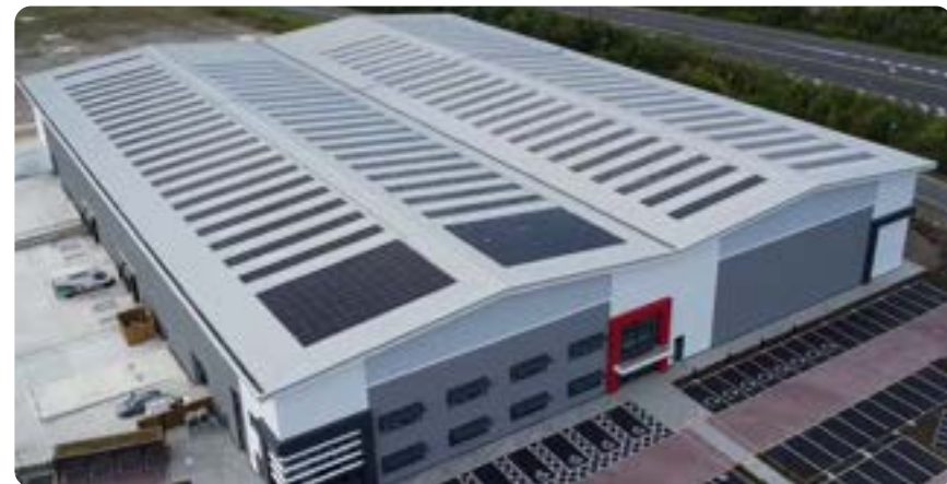
The new factory in Andover has been built with sustainability in mind and has been fitted with PV panels that will provide 397,000kwh per annum.
