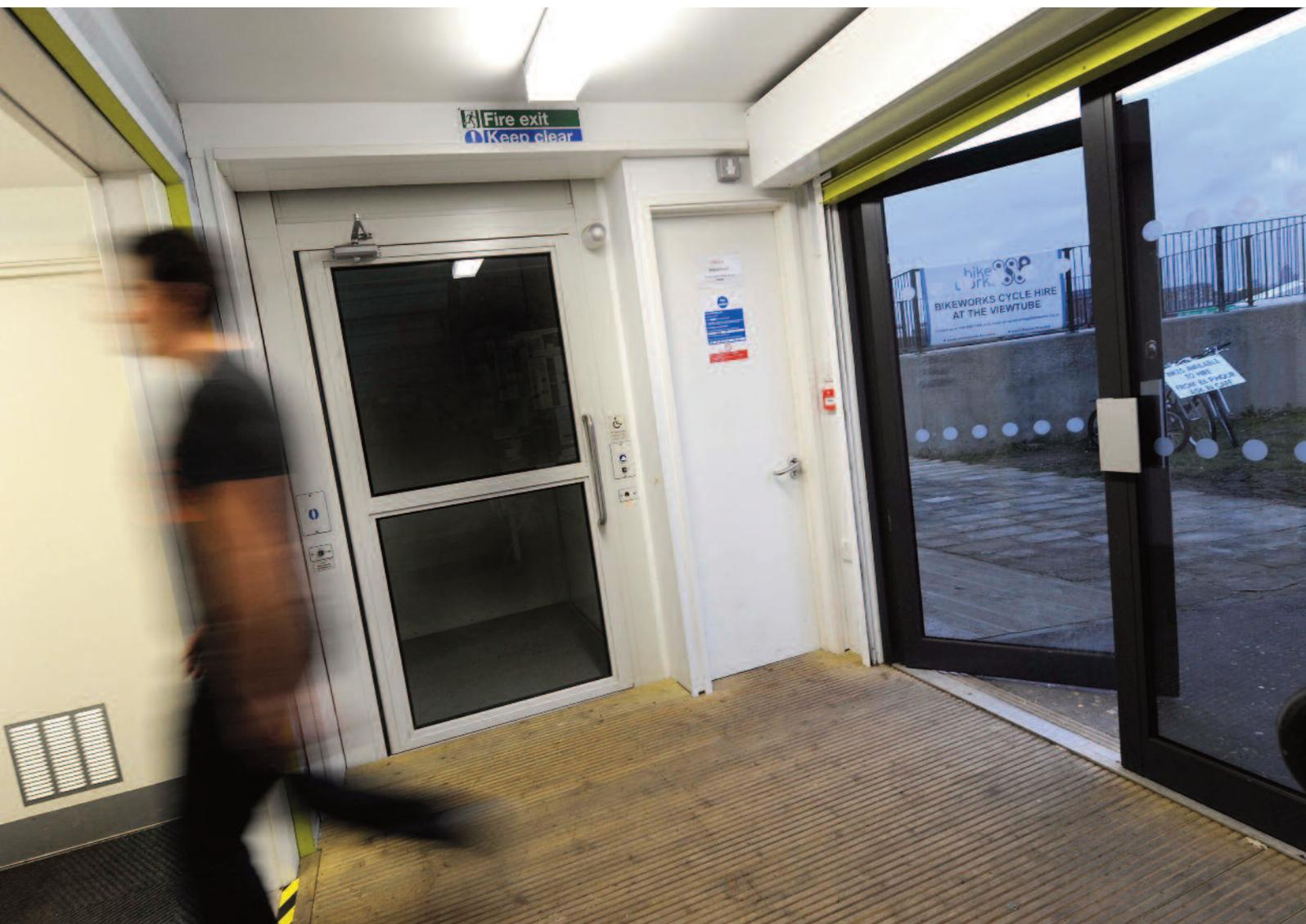
Supplied within a structure-supported enclosure, the Midilift SL does not require a purpose-built lift shaft or lifting beam, so installation was straightforward, taking just five days from fitting to commissioning. Simple and safe to operate it has a rated load of 400kg (4 persons). The platform is controlled by constant pressure buttons and has a maximum travel of 5m at a speed of circa 0.08m/s.
