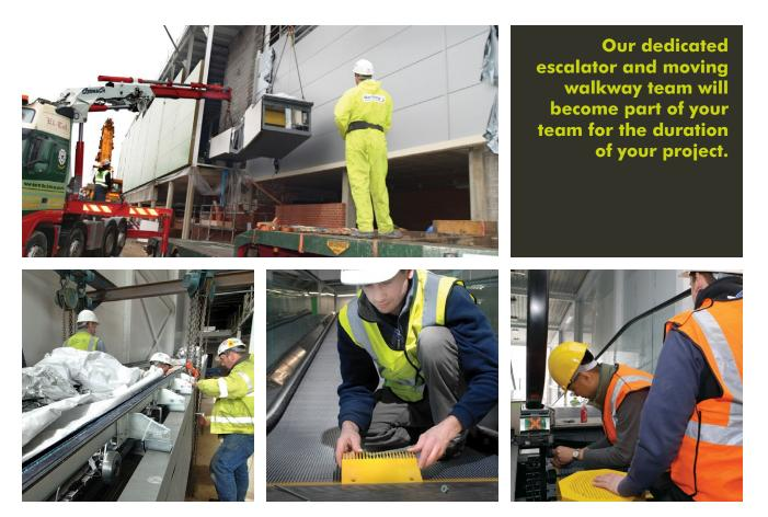
lifted and 'posted' through a purpose-built opening at retail level to be assembled alongside its permanent position. The process was repeated for the three remaining walkways but this time the assembly took place on the ground-floor car park level where the units were to provide fast access to the first retail floor.
