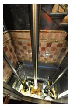
The direct-acting hydraulics use a telescopic ram to facilitate a reduced overall length to the piston that goes through the basement and into a small borehole (1470mm deep). Below this is Leicester Square station.
